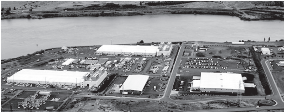
Figure 2.1 Photograph of Google's top-secret Dalles, OR data center, built near the Dalles Dam for access to cheap power. Note the large cooling towers on the end of each football-sized building on the left. These towers cool through evaporation rather than using more power-hungry chillers. Source: Melanie Conner, New York Times .
