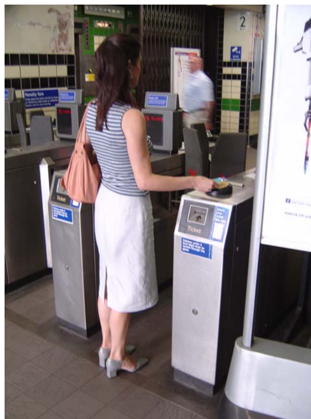
Fig. 1 Location of RFID units on entry gates: RFID readers have circular yellow reading areas. The entry slot for magnetic cards is also visible on the vertical surface of the gate
